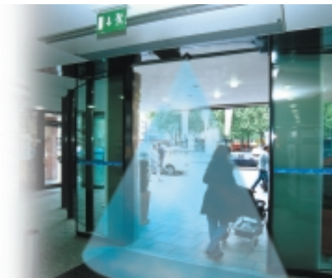
Sensing fields in accordance with lateral position of antenna Mounting height : 2.2 m Sensitivity : 6
